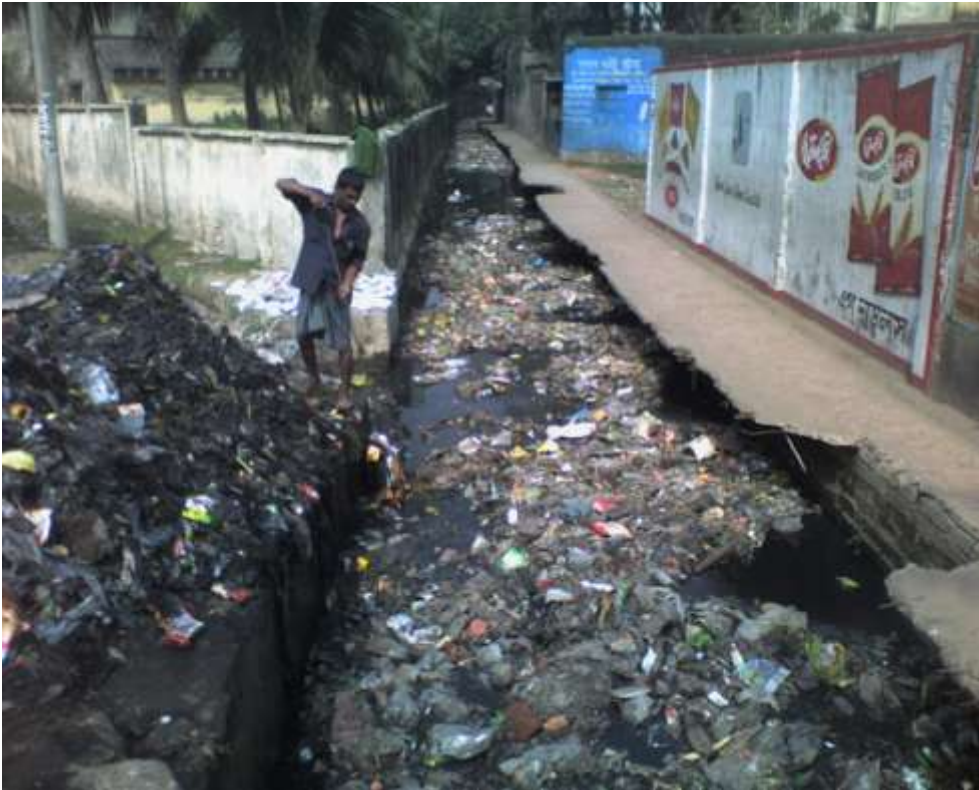
Picture: Dumping of city wastes into the drain has caused serious problems
