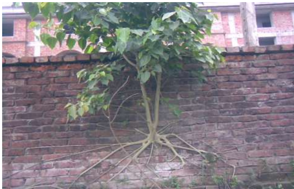
Picture: A banyan tree, anchoring roots on the wall without surface coatings
