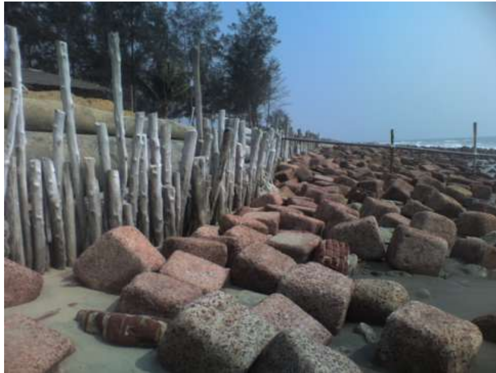
Picture: Wooden pilings and cement-concrete blocks to control sea beach erosion
